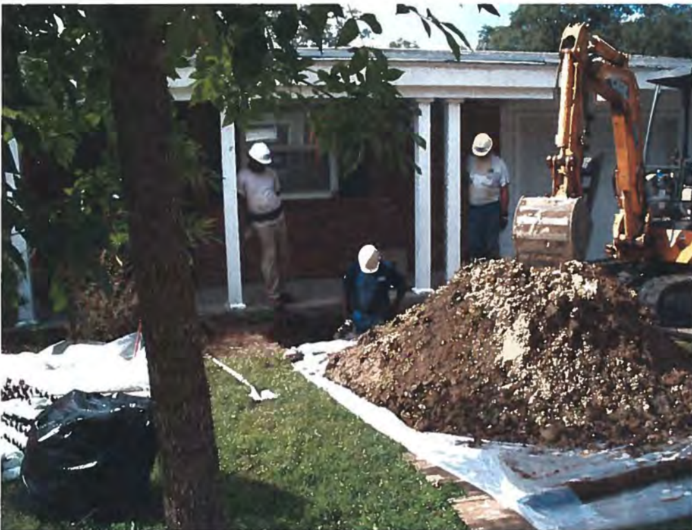
Picture 2: UST 310Ash removal in progress.
